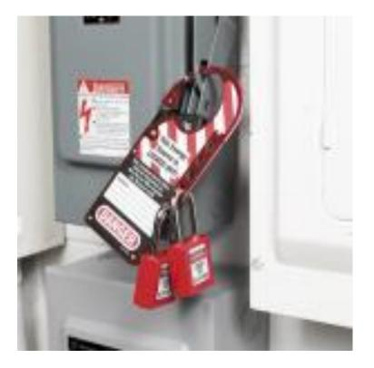
The above photograph shows an isolator locked out and two locks in place. Two or more locks are used when more than one person is working on the locked-out equipment.
